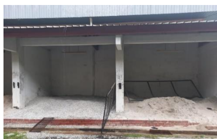
Figure 3.5 Coarse Aggregate at back of Brick Workshop
