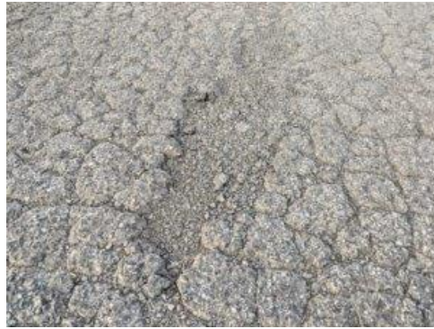
Rajah 2,10 pengikisan ravelling
