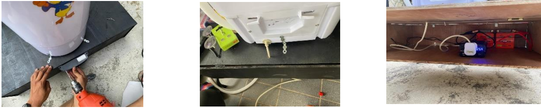
Figure 3.5.1.5 Installation of each material on the project framework
