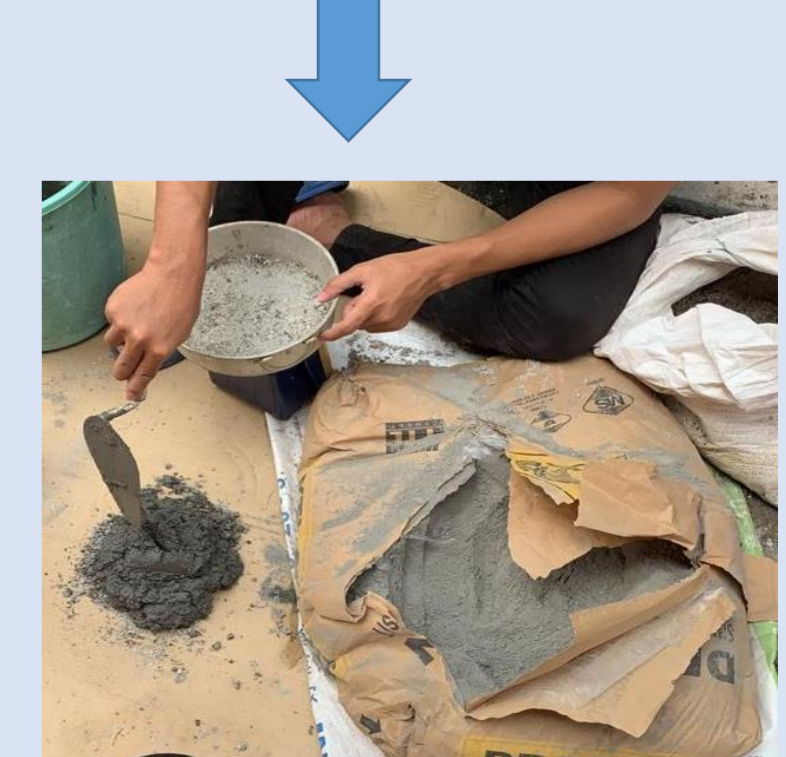
3) Mixing cement and sand
