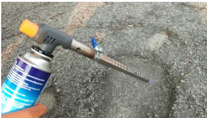
Figure 3.4.2.3: Make sure the pothole is dry
