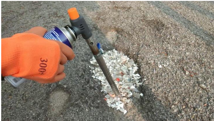
Figure 3.4.2.5: Melt the thermoplastics
