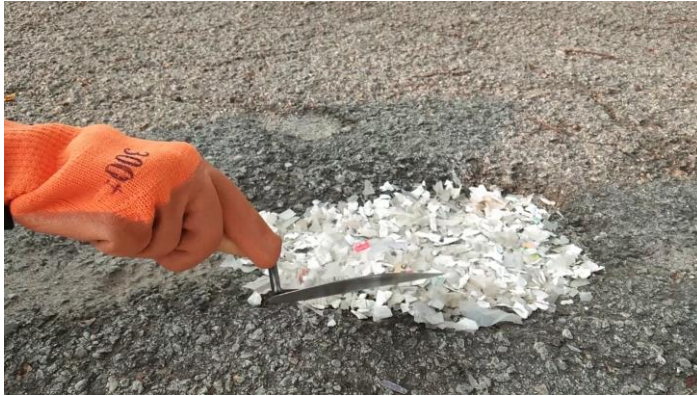
Figure 3.4.2.4: Spread the small pieces of thermoplastics into the pothole
