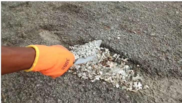
Figure 3.4.2.6: spread the aggregates on top of thermoplastic layers
