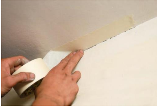
Figure 1.1 Attaching tape to the ceiling
