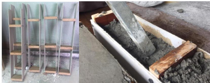
Figure 3.5: Pouring the mixture
