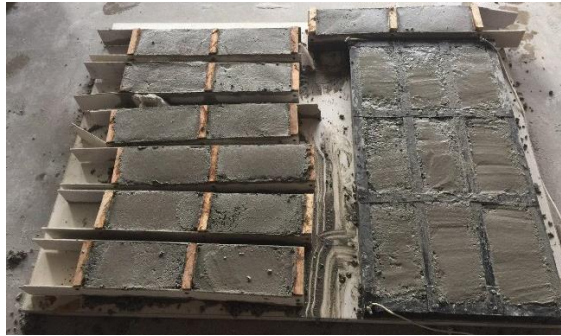
Figure 3.6: Flattened the brick surface
